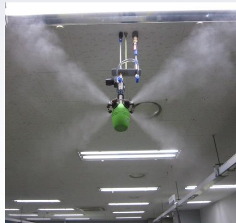
■ Ceiling type humidifying system
